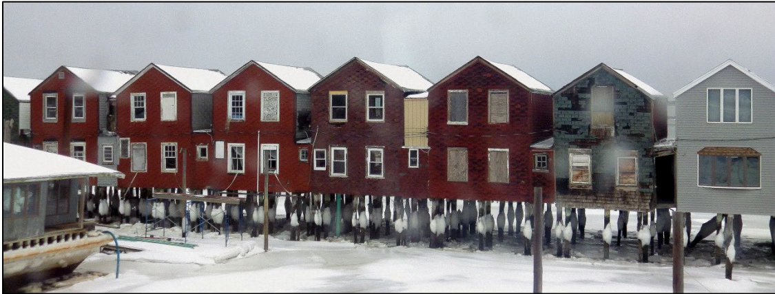
Figure 15: Photographs of the eligible properties near the Hammels high-frequency flood risk reduction: New York City Transit System building (top), 2 Beach 85 th Street (middle) and the Hammels Pier (bottom) (NYSHPO CRIS 2019).
